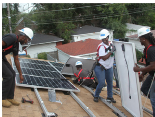
Figures 12 & 13. Workers installing solar panels. Image credit: Elevate.
