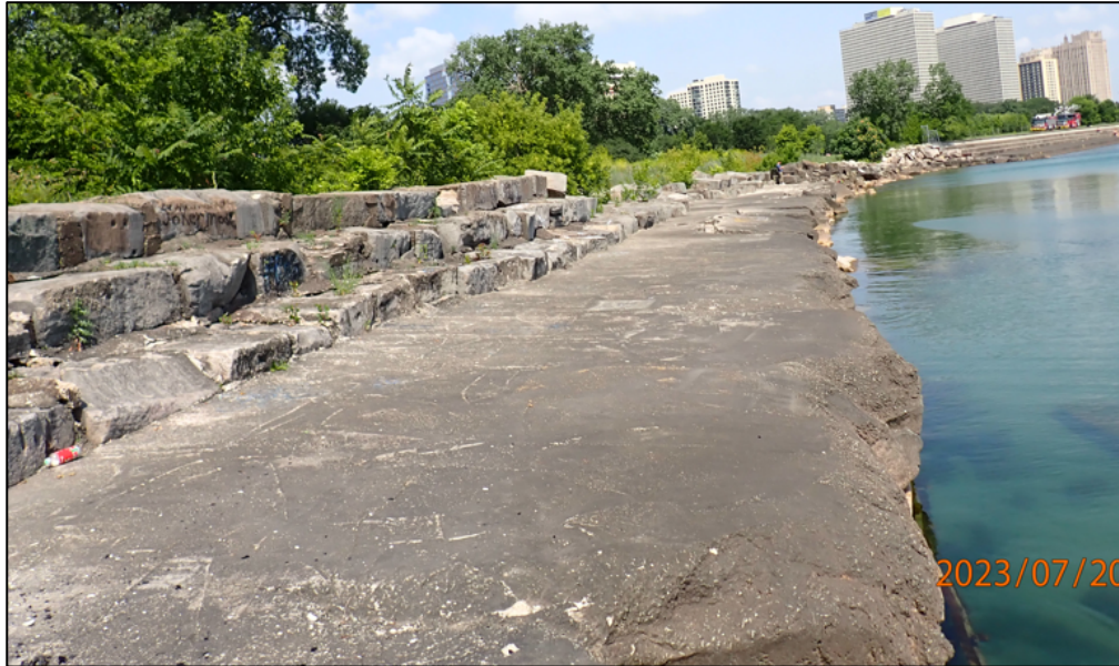
Figure 5.13. Terrestrial View of S5
