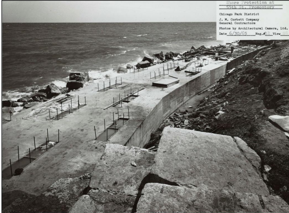
Figure 2.6. Construction of the Concrete "Coffins" atop the Concrete Platform
