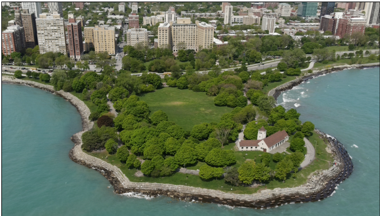
Figure 2.1. Overall View of Promontory Point, Looking West (May 2023)
