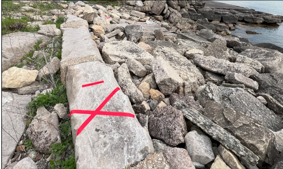
Figure 5.16. Terrestrial View of S6
