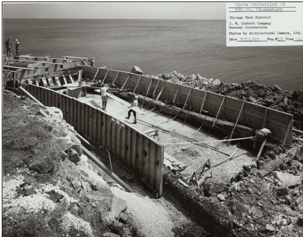
Figure 2.5. Construction of Concrete "Coffins" on the Northeast Shore of the Peninsula
