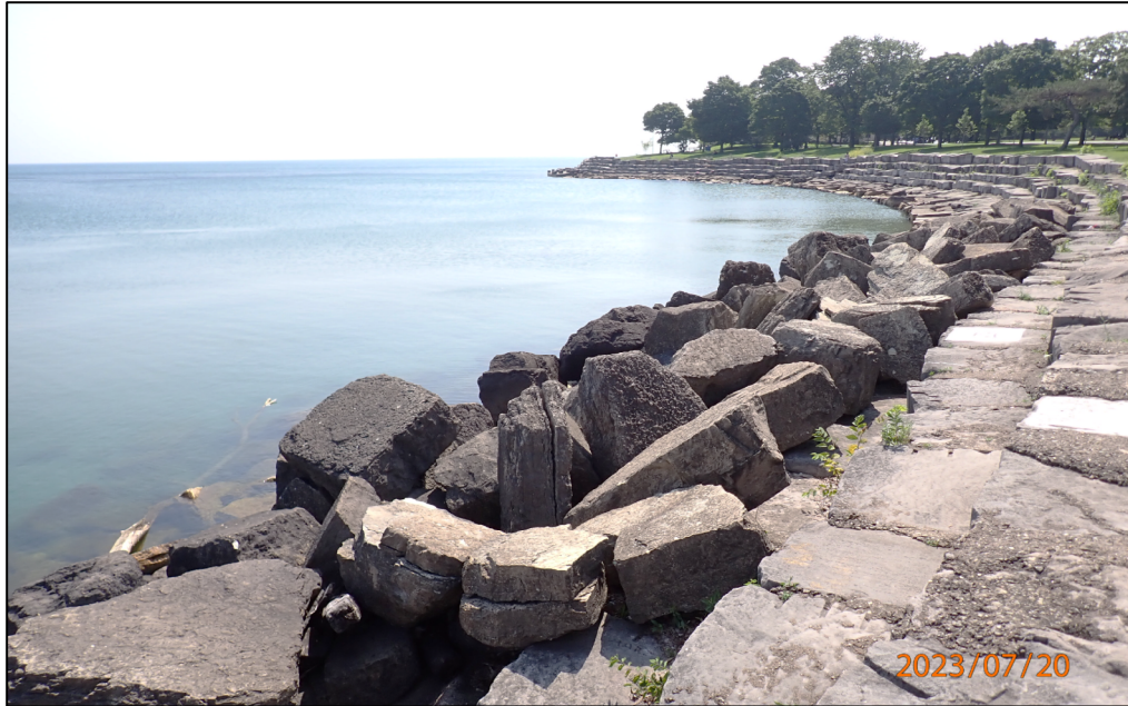
Figure 5.10. Terrestrial View of S4
