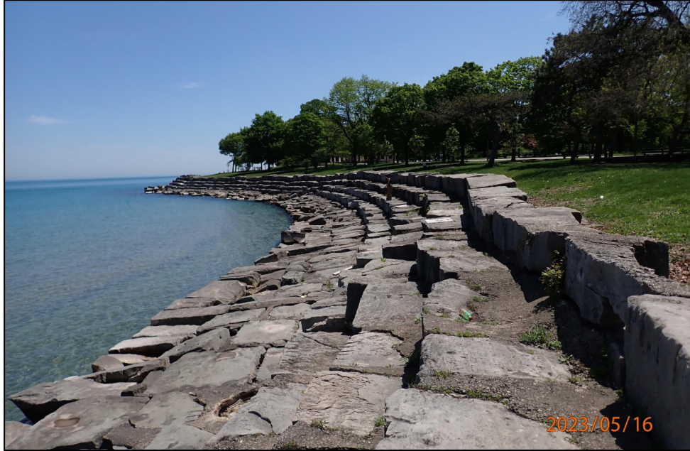
Figure 5.7. Terrestrial View of S3
