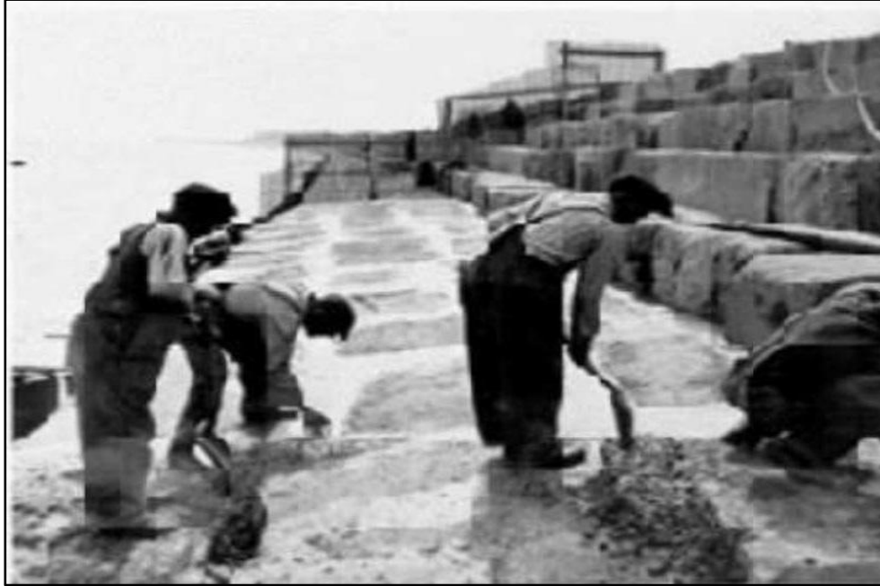
Figure 2.4. Construction of the Limestone Structures at Promontory Point
