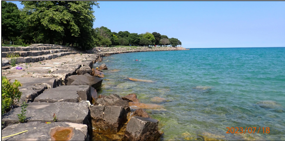
Figure 5.1. Terrestrial View of S1
