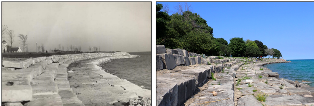
Figure 3.1. Historic (left) and Present-Day (right) View of the Limestone Revetment with Limestone Promenade
