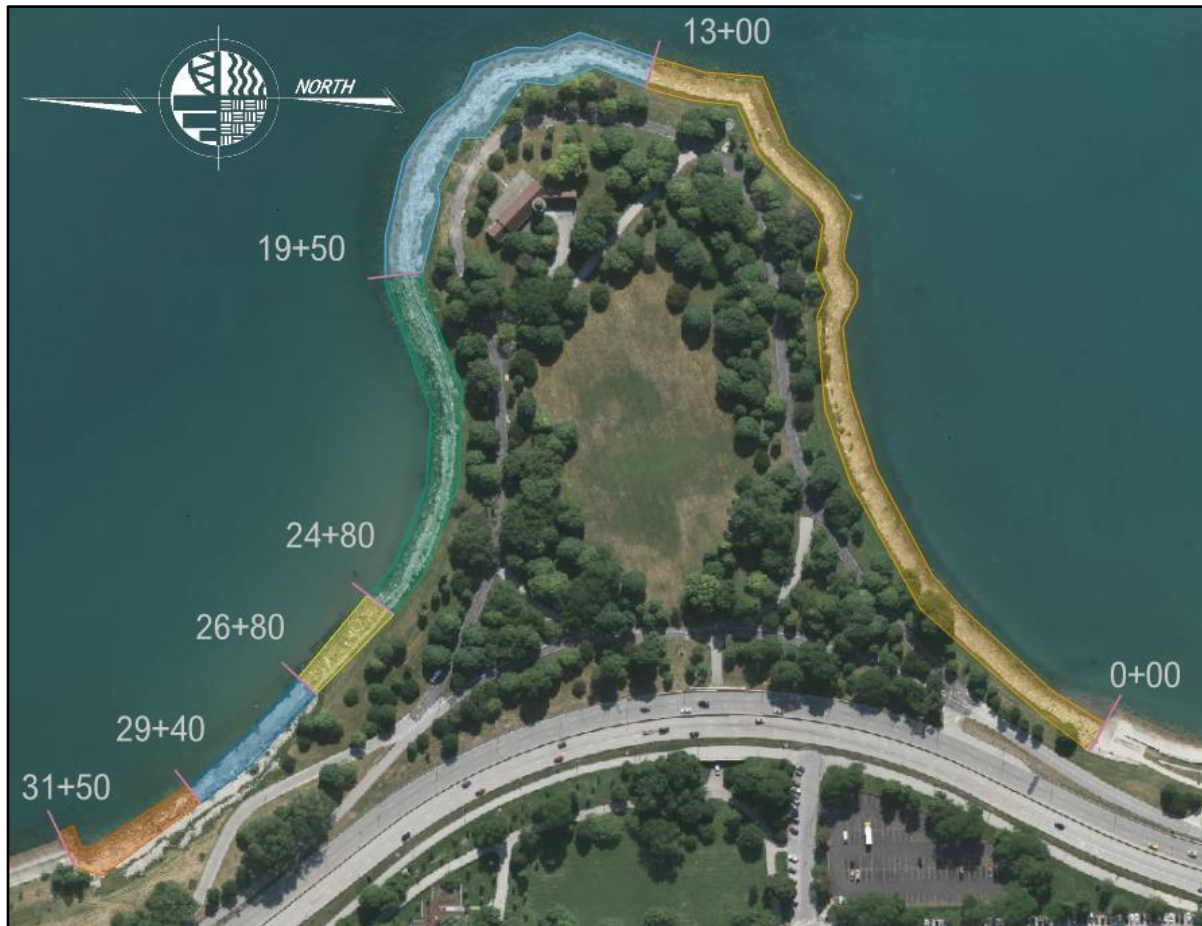
Figure 1.1. Overview of Promontory Point Sections, Section 1 through Section 6 1
