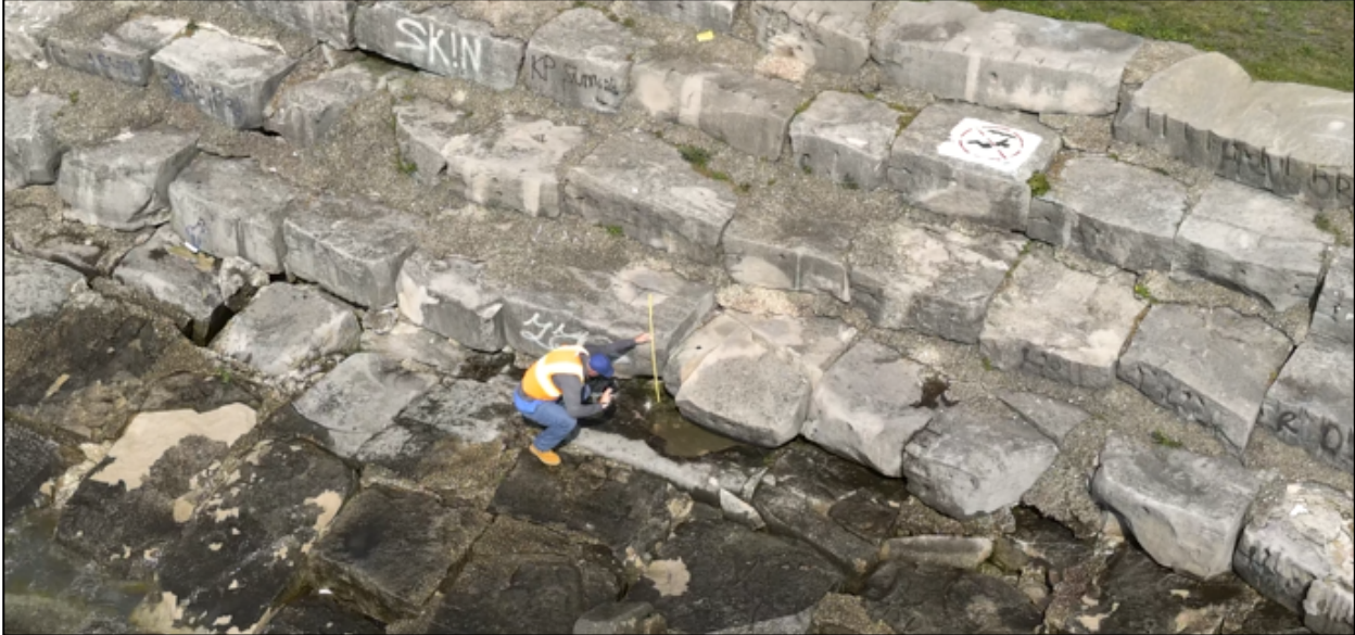
Figure 3.2. View of Engineer Measuring Limestone Block Height during the Above-Water Inspection
