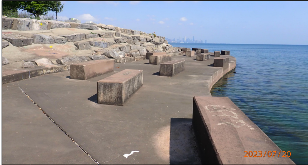
Figure 5.4. Terrestrial View of S2
