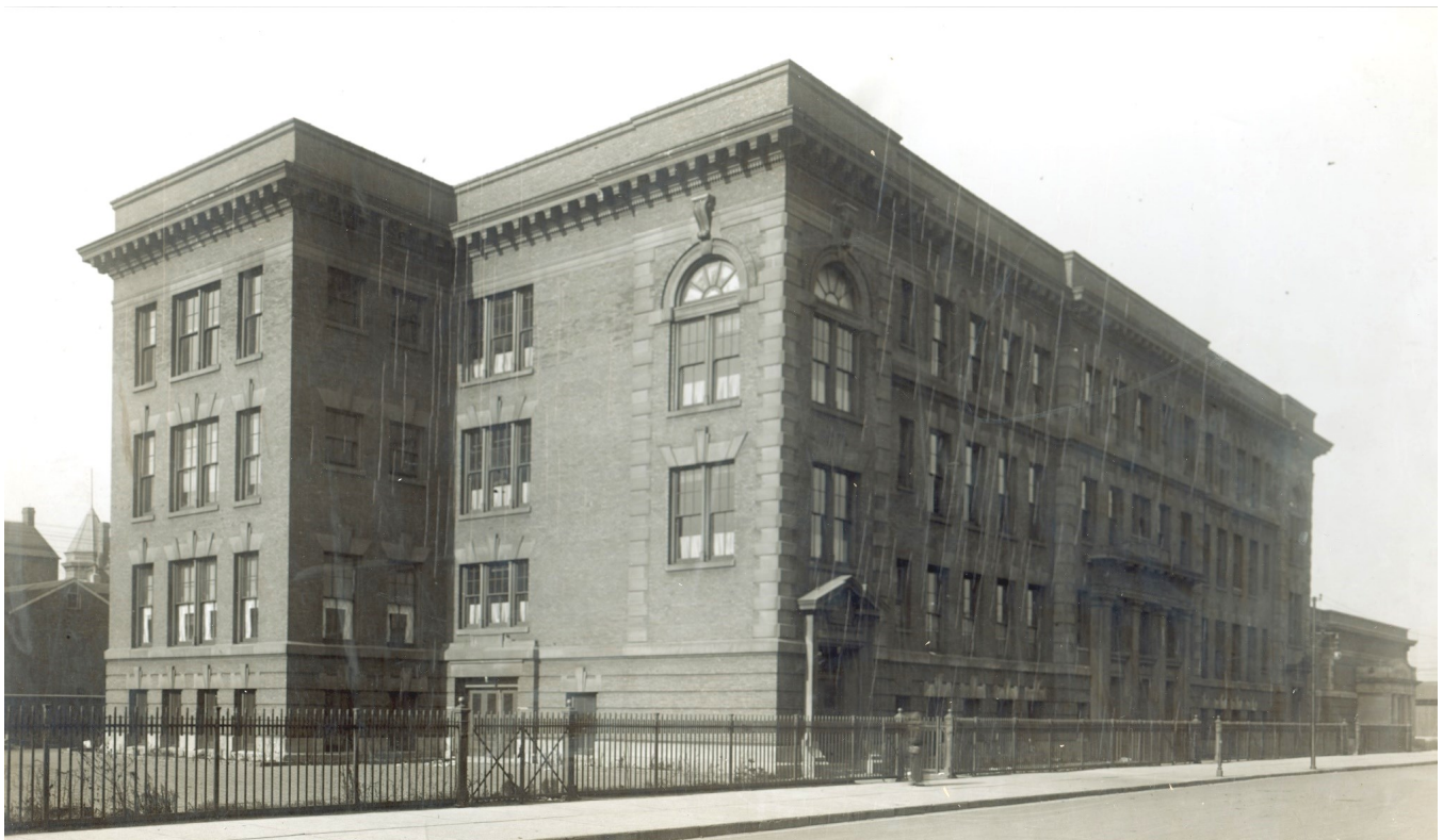
Top : Designed by architect August Fiedler in 1890, the Komensky School (now Perez School Annex 2001 S Throop St.) was named in honor of a Czech philosopher. The design of the building incorporates rectilinear forms of red brick, with a substantial rusticated limestone stone base.
