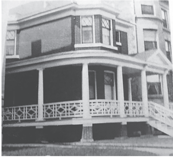
Fig. 1. Jesse Binga's house at 5922 South Park Avenue. The Bingas bought this redbrick house in 1917. (South Park Avenue was originally named Grand Boulevard, then it became South Park Avenue, then South Parkway, and today it is Dr. Martin Luther King Jr. Drive.) PHOTOGRAPH COURTESY OF CAROLYN LOUISE DENT-JOHNSON.
