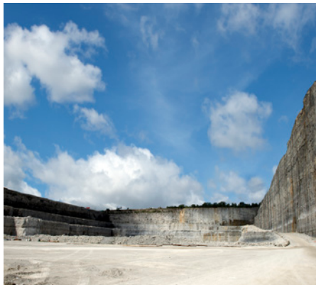
The 7.9 billion gallon Thornton Reservoir, part of the Calumet TARP system.
