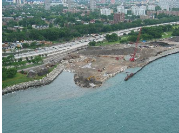
Photo of construction at 39 th Street (2003)
