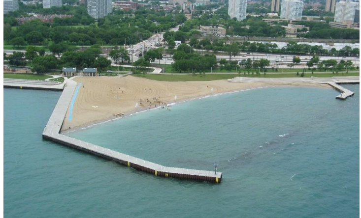
Photo of Completed 31 st Street Beach (2003)
