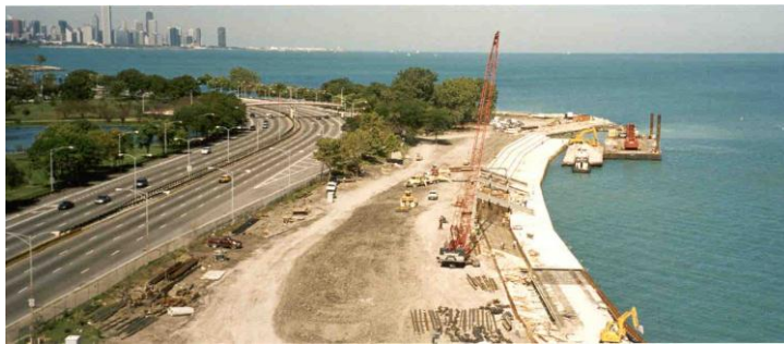
Photo of construction at 51 st Street (2000)
