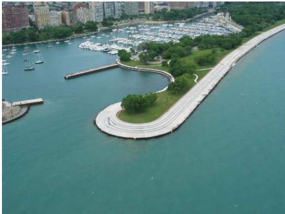
Photo of Completed Belmont Harbor (2003)
