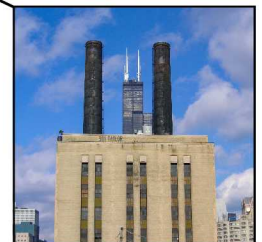
Union Station Power House
