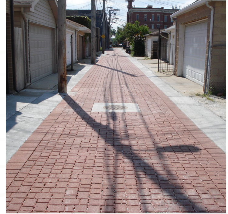
Dedicated funding through Chicago's Capital Bond program has allowed CDOT to accelerate the pace of green alley installation across Chicago. Credit: Chicago Department of Transportation
