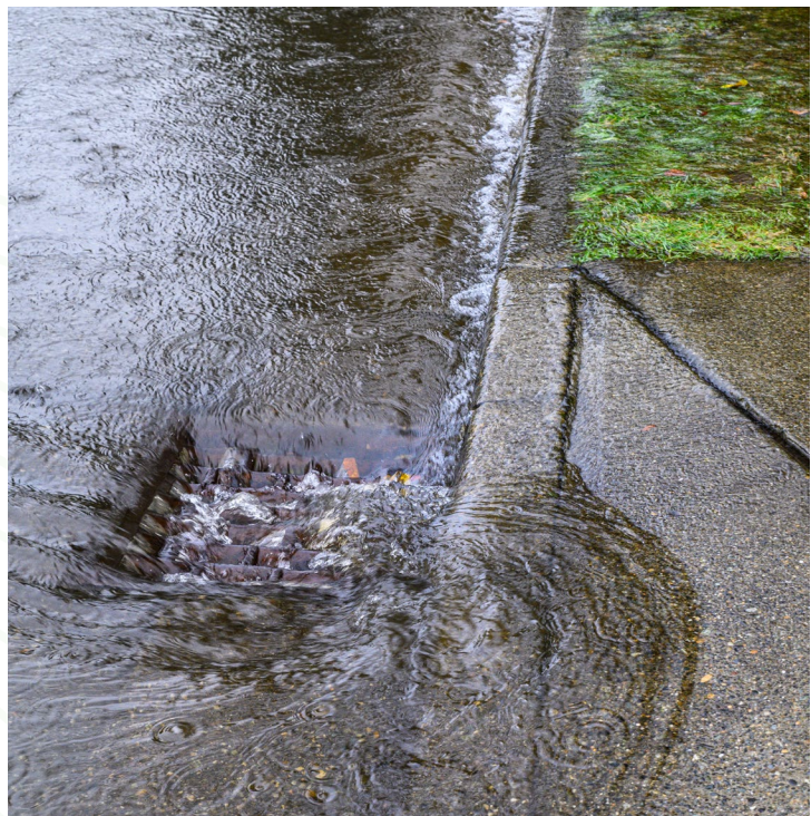
Water from heavy rainfall flows into the sewer.
