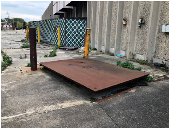
15 LOADING BAY - NORTH (NO HYDRAULICS OBSERVED)
