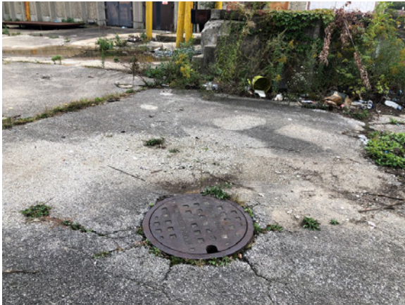
9 SEWER COVER - NORTH
