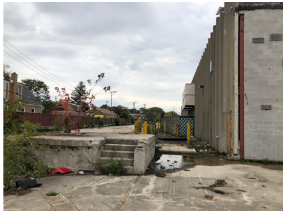
28 WEST ADJOINING - LOADING DOCK
