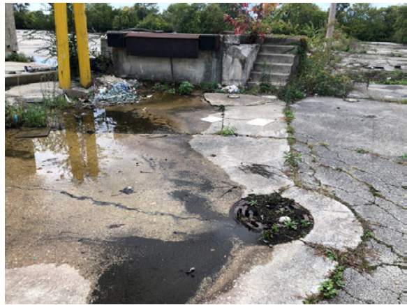
12 STORM WATER - NORTH
