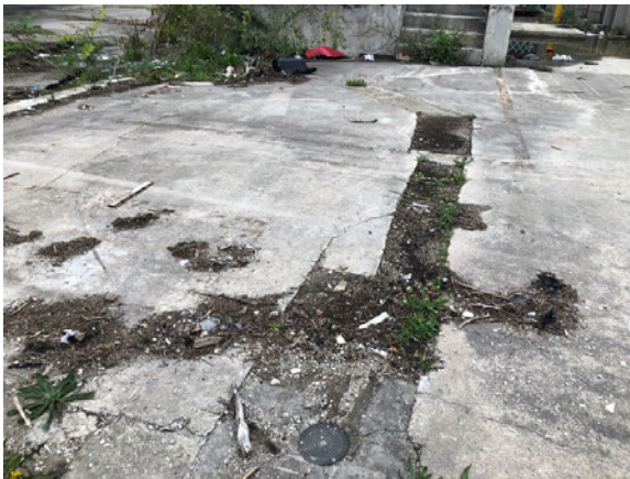
29 WEST ADJOINING - LOADING DOCK
