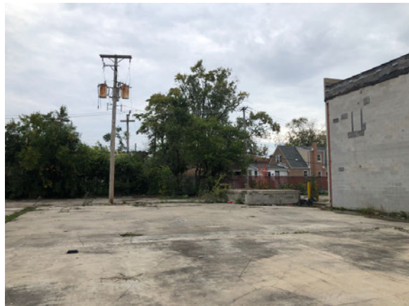
30 TRANSFORMER - NORTHWEST ADJOINING
