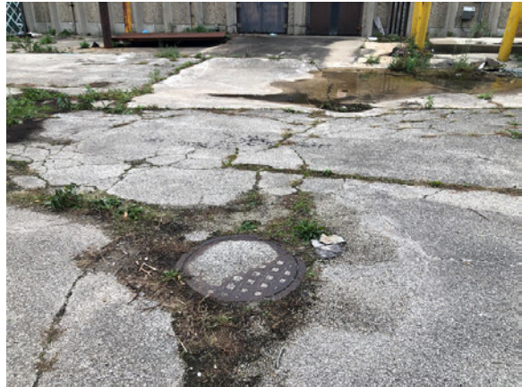
10 SEWER COVER - NORTH
