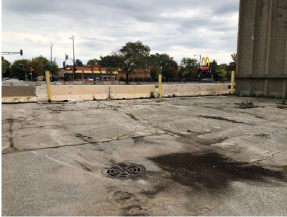
13 STORM WATER - NORTH
