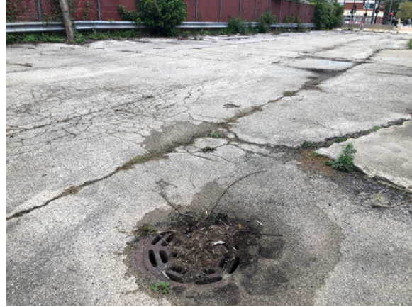
14 STORM WATER - NORTH
