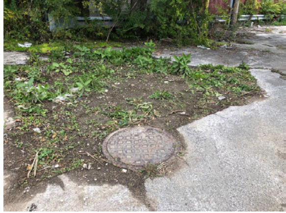
8 SEWER COVER - NORTHWEST
