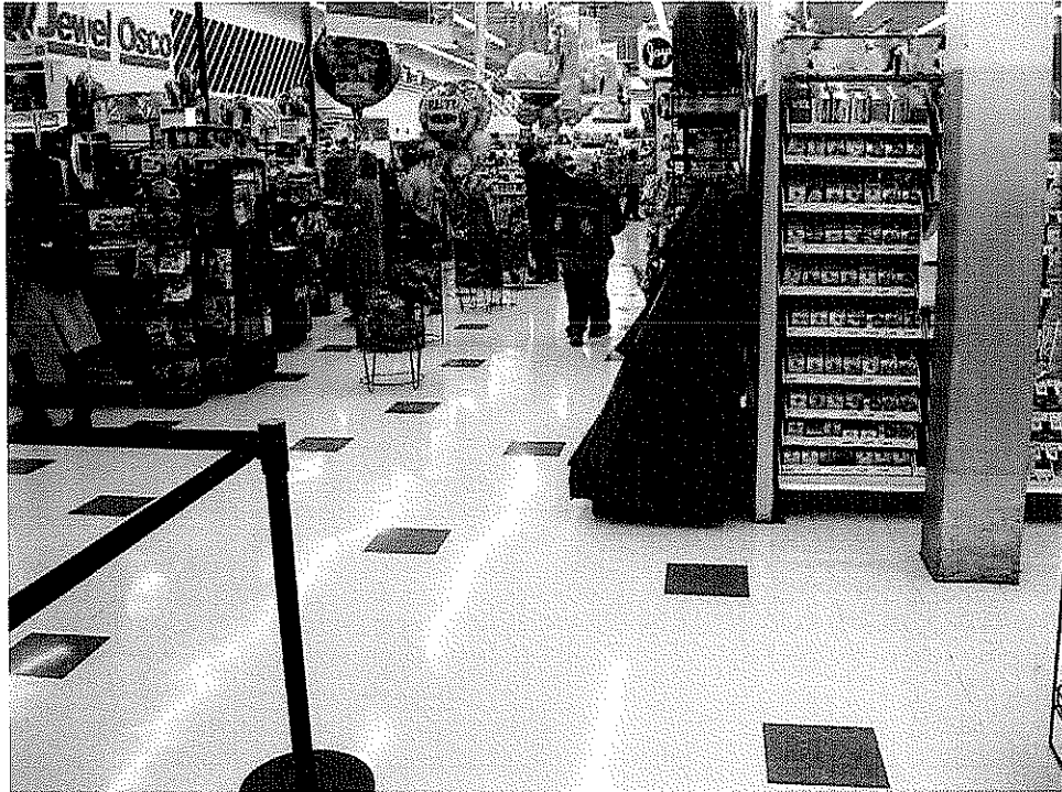
View of the 12"x 12" white pattern floor tile and the 12"x12" blue accent floor tile located in the main sales area.
